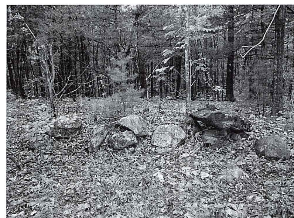
VIEW A - LOOSELY PLACED STONES INDICATIVE OF CHARACTER OF WALLS IN PROJECT AREA (SEE PLAN BELOW FOR LOCATION)
