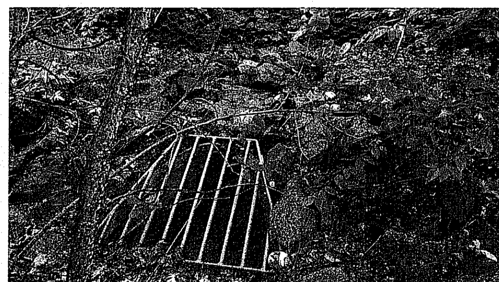
4 EXISTING 18"Ø CULVERT ADJACENT TO SAND FILTER #1 NOT TO SCALE
