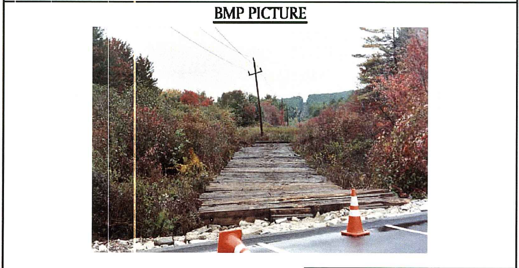
CM-3 CONSTRUCTION MAT LAYOUT (WITH TRANSITION) APPROVED BY: VICE PRESIDENT, ENVIRONMENTAL SERVICES PRINTED COPIES ARE NOT DOCUMENT CONTROLLED. FOR LATEST AUTHORIZED VERSION PLEASE REFER TO THE NATIONAL GRID ENVIRONMENTAL INFONET SITE.
