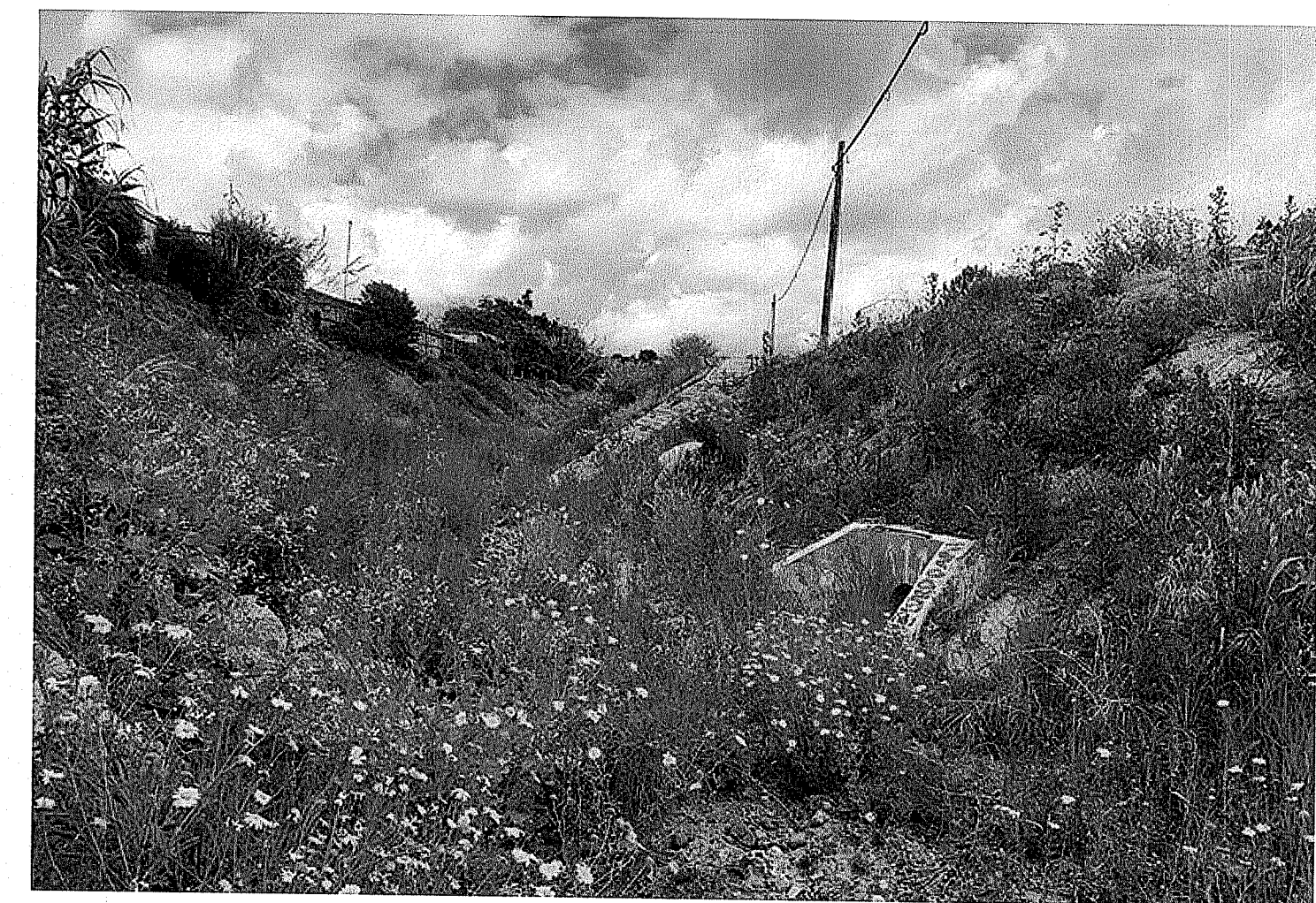
FIGURE OF REVEGETATED BANKS ARMORED WITH PROPEX PRODUCTS
